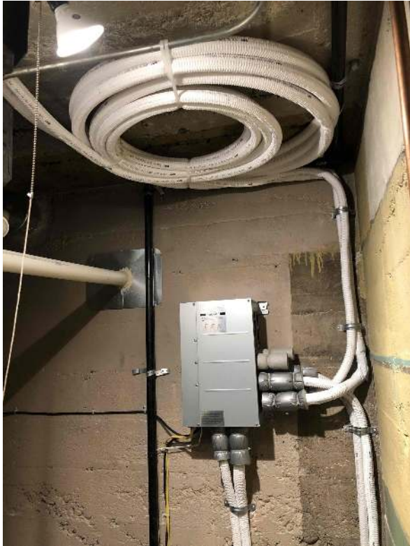
Line Set and Branch Box | S9v2 Furnace with Intelli Heat Dual Fuel Coil
