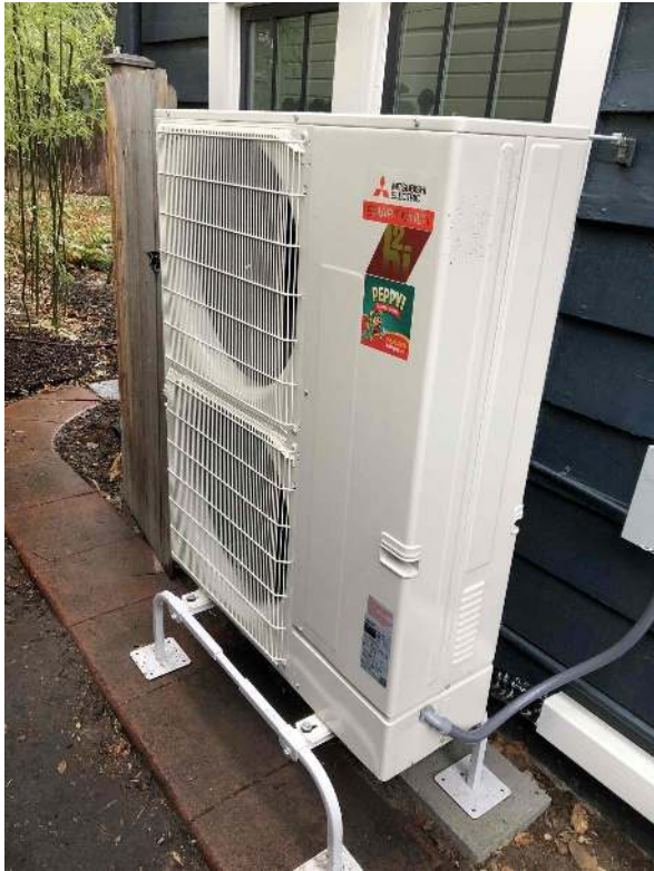
Hyper Heat Outdoor Multizone Unit | Indoor GL Wall Mount Head Bdrm
