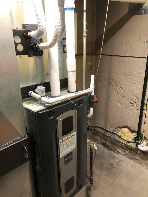
Line Set and Branch Box | S9v2 Furnace with Intelli Heat Dual Fuel Coil
