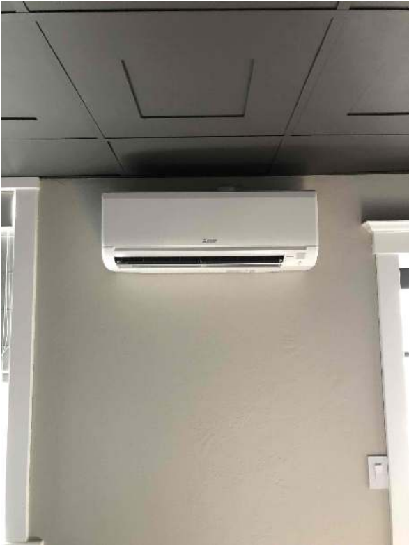
Hyper Heat Outdoor Multizone Unit | Indoor GL Wall Mount Head Bdrm
